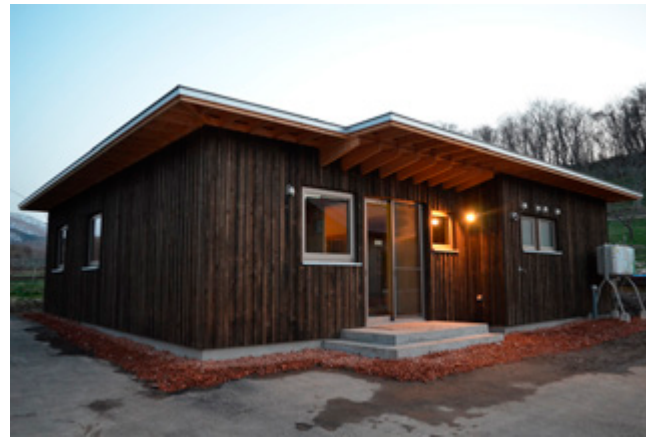
The shared house used as the base for the assessments
